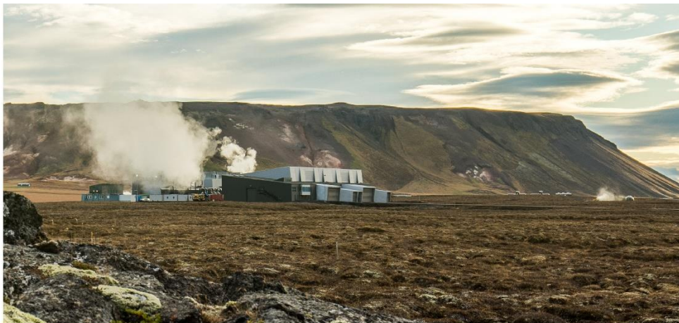
Figure 5: Theistareykir power plant. Photo: Mannvit.
