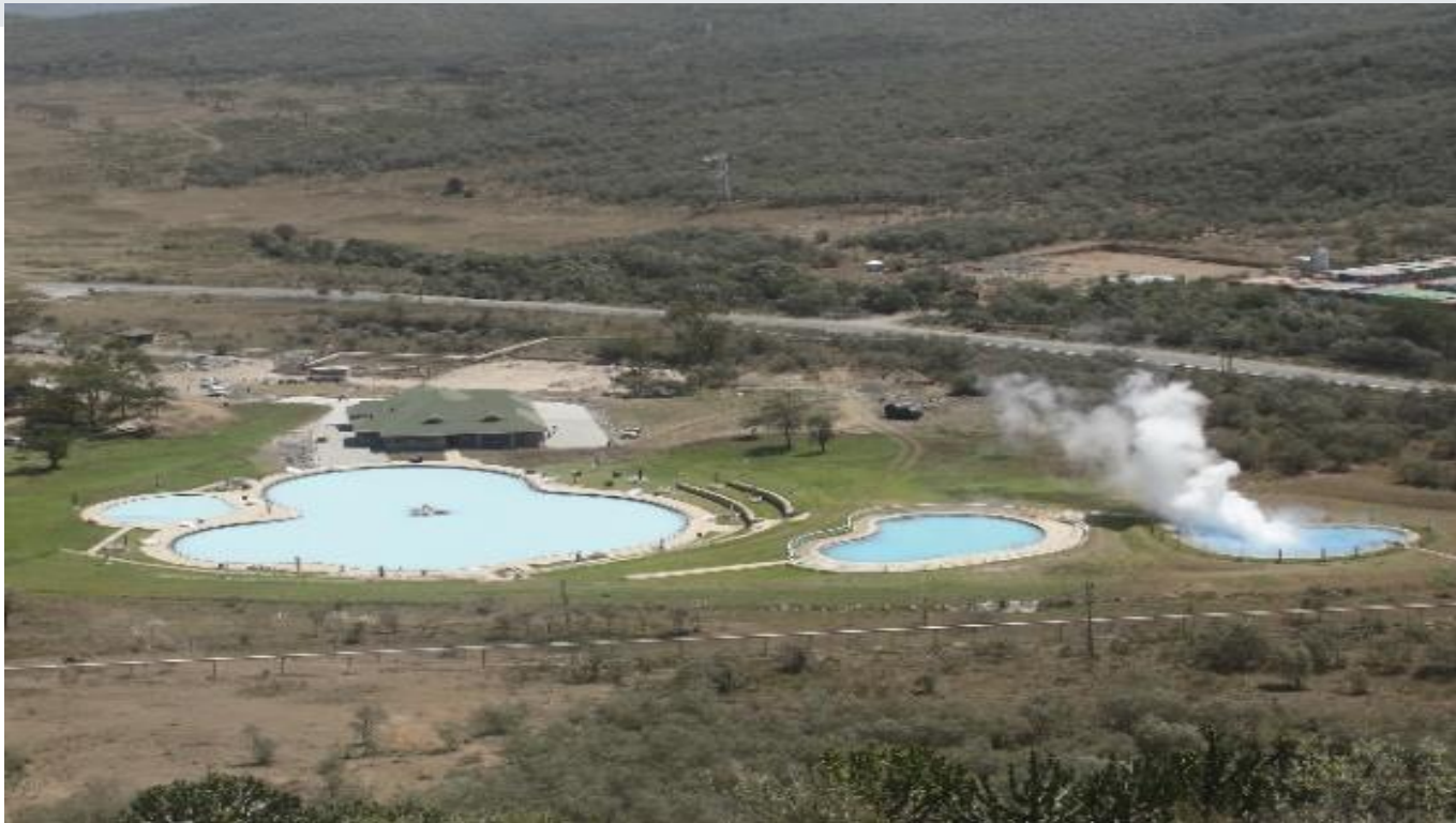
Panoramic view of the Olkaria Geothermal Spa
