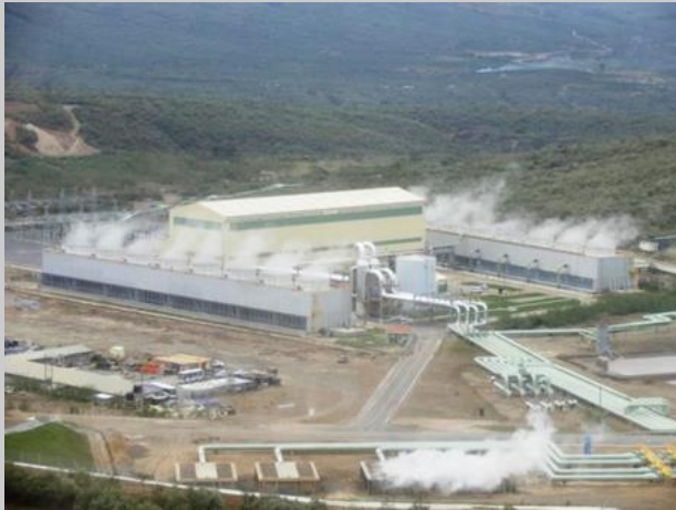
Olkaria IV 2 x 70 MW single flash plant (Toshiba, 2015)
