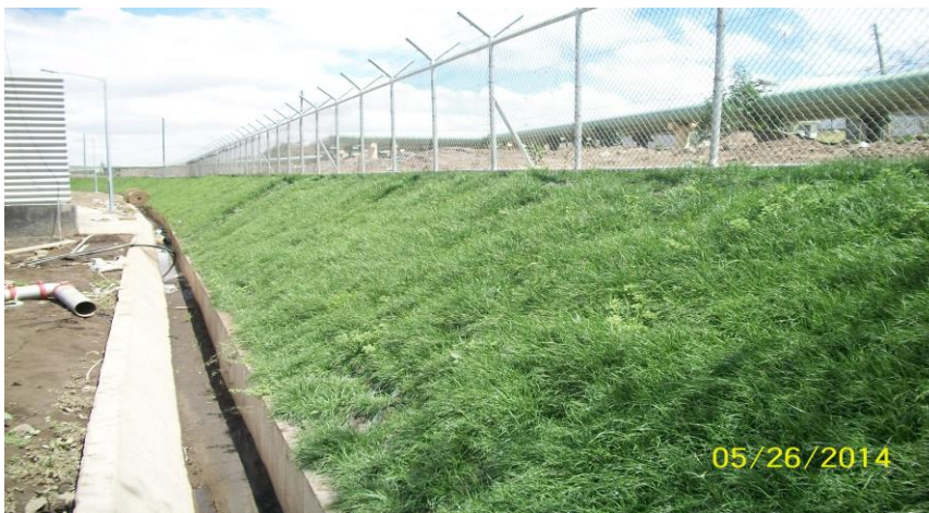
Plate 1: Photo Showing Grass Planted at Olkaria IV site Using Hydro Seeding Technology
