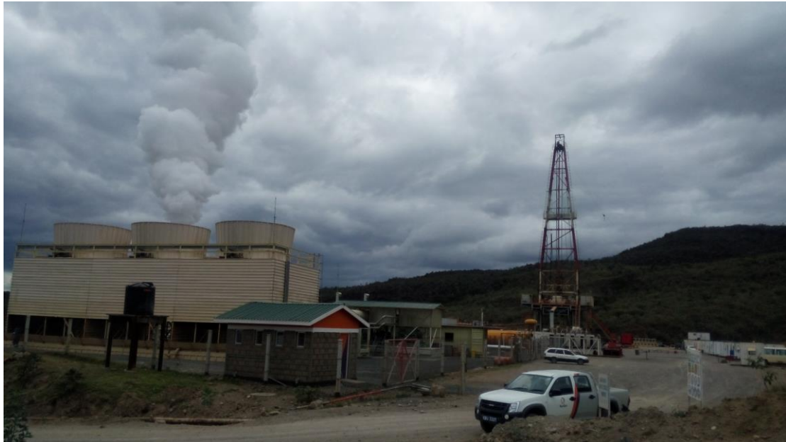
Figure 2. Wellhead OW-37 with rig KGN02 drilling on the same pad
