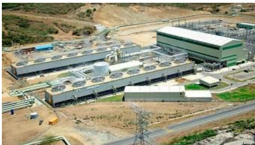
Figure 1: Olkaria 1 Additional Units aerial view
