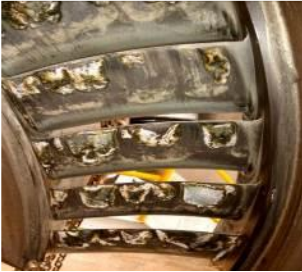
Figure 10: 1 st stage stationary nozzle silica scaling
