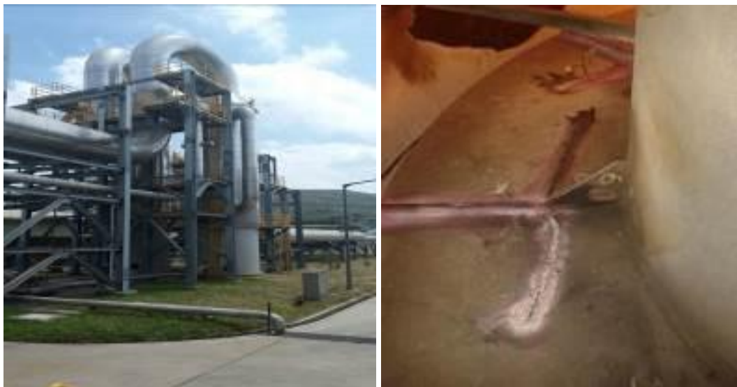
Figure 8: Steam scrubber and internal repairs
